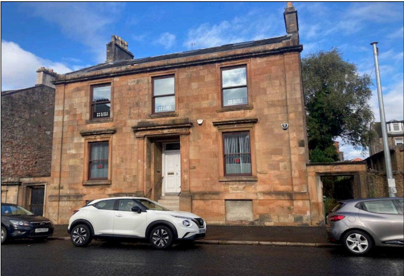
View of the front elevation of 20a Union Street, Greenock.
