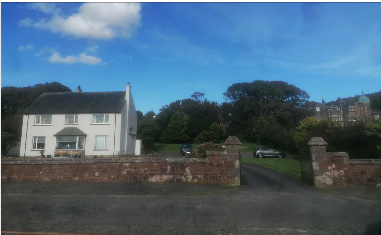
View of site looking north from Wemyss Bay Road. Ardvaar is the house on the left and the Category 'B' listed Dunloe is on the right.
